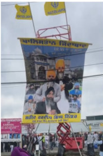
The big banner also guarded wires and scissor lift from falling on the ground
