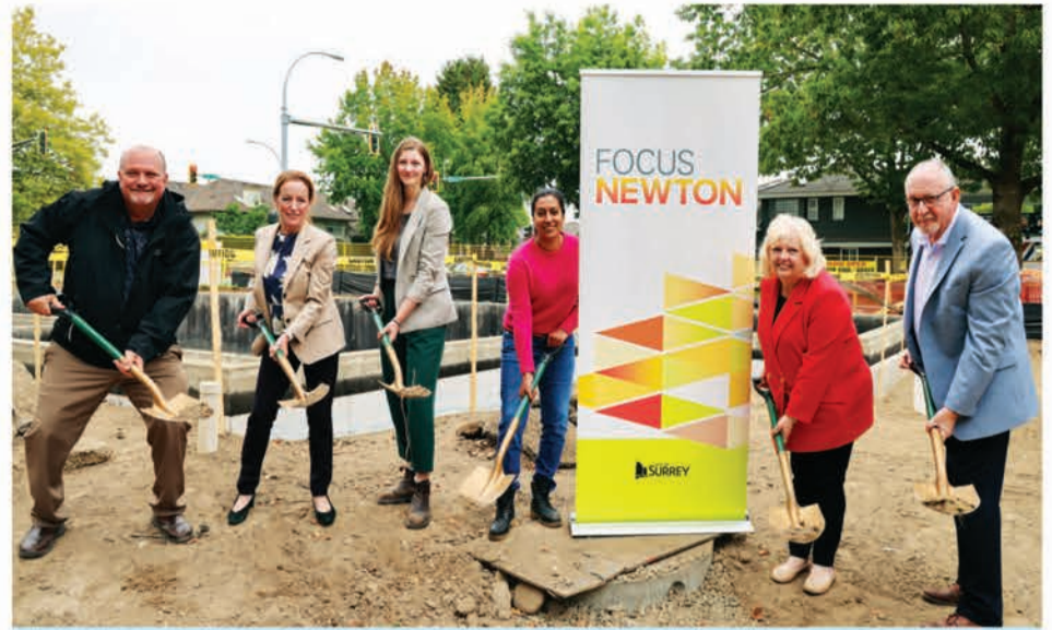
Mayor Brenda Locke, members of Surrey City Council and architect Natalie Copping from 04Architecture celebrate the groundbreaking of the Strawberry Hill Community Hall on Sept. 12 in Newton.
